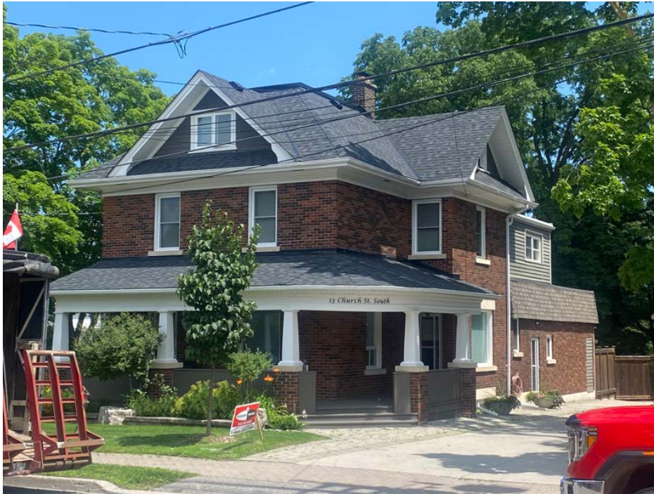
Figure 7 Photograph of the Graham-Young House's front (west) and south elevations, looking northeast from Church Street South. Note the house's complex form and roof composition, mottled rugged brick cladding, shingle-clad gables, flat headed windows and doors, and the large curved wraparound verandah on the front (west) elevation. (Source: HUD, 2024).
