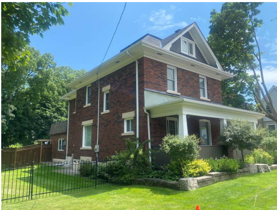
Figure 8 Photograph of the Graham-Young House's front (west) and north elevations, looking southeast from Church Street South (Source: HUD, 2024). Note the house's mottled rugged brick cladding, shingle-clad gables, flat headed windows and doors with stone sills and/or lintels, and the large curved wraparound verandah on the front (west) elevation. (Source: HUD, 2024).
