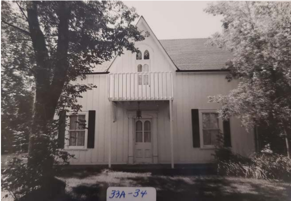
Figure 3 1984 photograph of the Horner House at 11644 Leslie Street, showing the building's front (east) elevation. Note the building's 1 ½ storey massing, side gable roof with front gable, symmetrical front façade, and top-storey rounded doorway with paired lancet arch transoms. Also note the building's balcony and paneled front door with round-arched lites and classical door surround, which have since been removed. (Source: LACAC)
