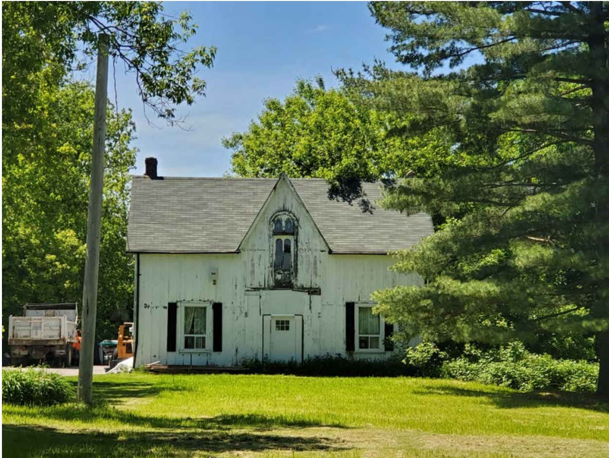
Figure 4 Current photograph of the Horner House at 11644 Leslie Street, showing the building's front (east) elevation. Note the building's 1 ½ storey massing, side gable roof with front gable, symmetrical front façade, and top-storey rounded doorway with paired lancet arch transoms. (Source: HUD 2024)
