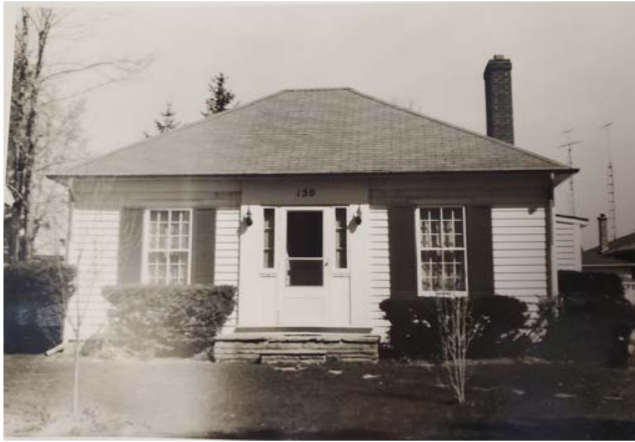
Figure 3 1978 photograph of the Thomas Smith House 159 Mill Street. Note the structure's one storey massing, frame construction, medium-sloped hipped roof, symmetrical three-bay front façade, central doorway with half-sidelights, and 12-over-12 windows. (Source: Richmond Hill LACAC)
