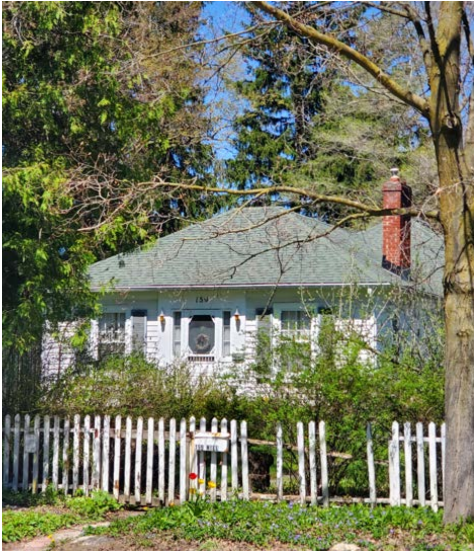
Figure 5 Current photograph of the Thomas Smith House at 159 Mill Street looking north, showing the structure's front (south) elevation. Note the structure's one storey massing, frame construction, medium-sloped hipped roof, symmetrical three-bay front façade, central doorway with half-sidelights, and 12-over-12 windows. (Source: HUD 2024)
