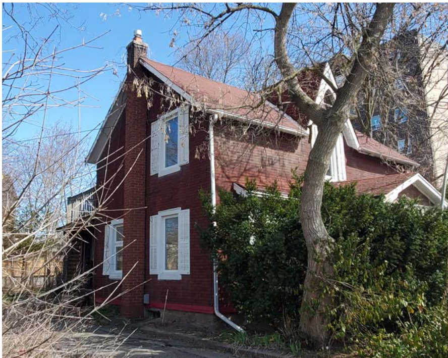
Figure 8 Current photograph of Maple Villa at 55 Richmond Street facing northeast, showing the west elevation. Note the 1 ½-storey massing, front gable, and flat-headed windows with stone sills and wood surrounds. (Source: HUD 2024)
