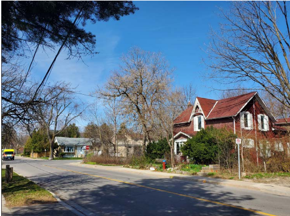
Figure 9 Current photograph of Maple Villa looking northwest, showing the structure's village core context on Richmond Street. Note the surrounding fine-grained residential streetscape along Richmond Street. (Source: HUD 2024)
