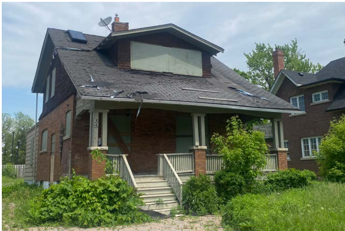
Figure 10 Current photograph of the subject property looking northeast, showing the principal (south) and west elevations. Note the house's rectangular plan and 1 ½-storey massing, the low-pitched side-gabled roof with a large, central gabled dormer, the brick and shingle cladding, exposed rafter tails, and the full-width front porch supported by grouped square columns on brick pedestals. (Source: HUD, 2024)
