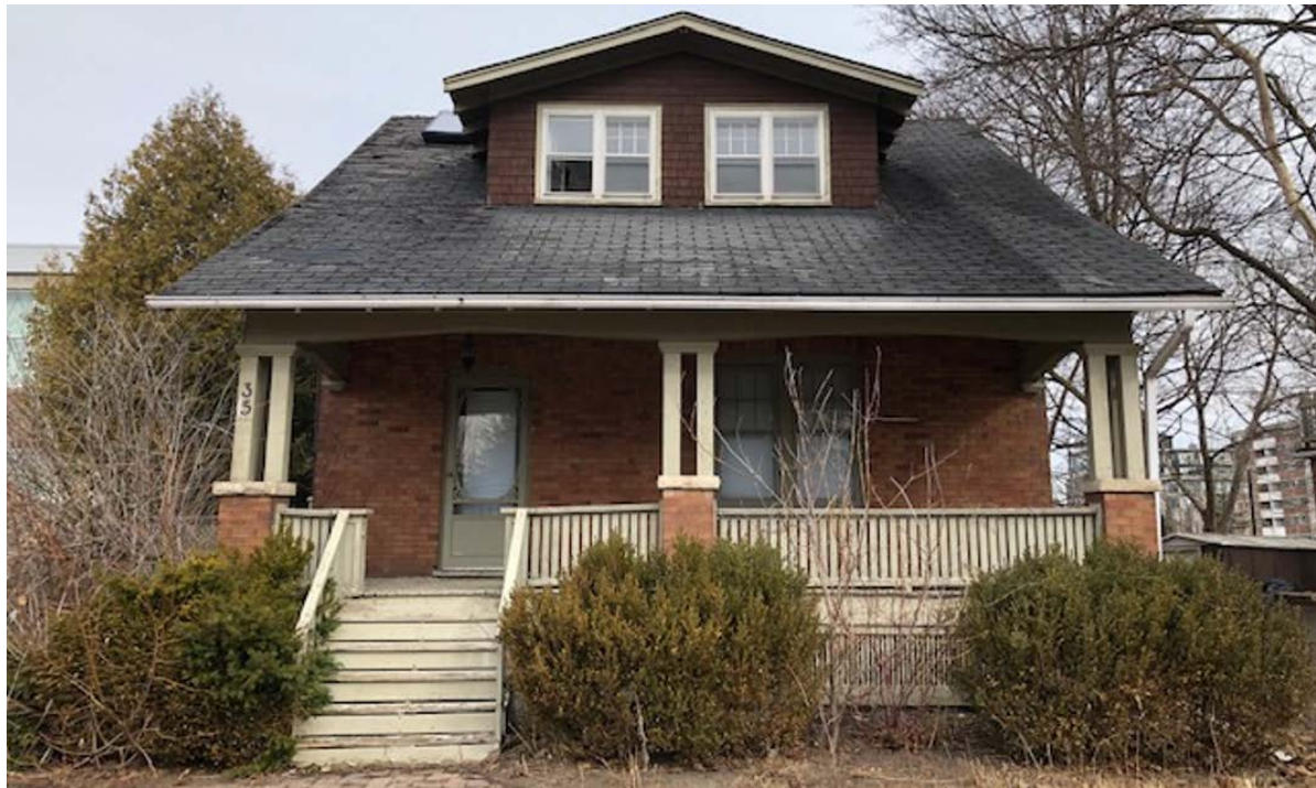
Figure 9 2021 photograph showing the subject property at 35 Wright Street prior to all windows and doors being boarded up for safety reasons. Note the period wood six-over-one window units and glazed front door. (Source: HUD, 2021)
