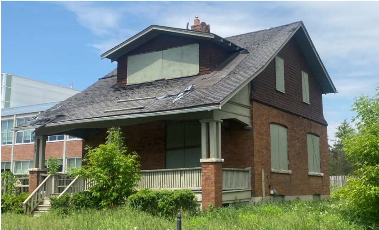
Figure 11 Current photograph of the subject property looking northwest, showing the principal (south) and east elevations. Note the house’s rectangular plan and 1 ½-storey massing, the low-pitched side-gabled roof with a large, central gabled dormer, the brick and shingle cladding, exposed rafter tails, and the full width front porch supported by grouped square columns on brick pedestals. (Source: HUD, 2024)
