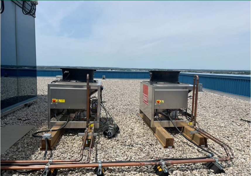
EBC HVAC Replacements
