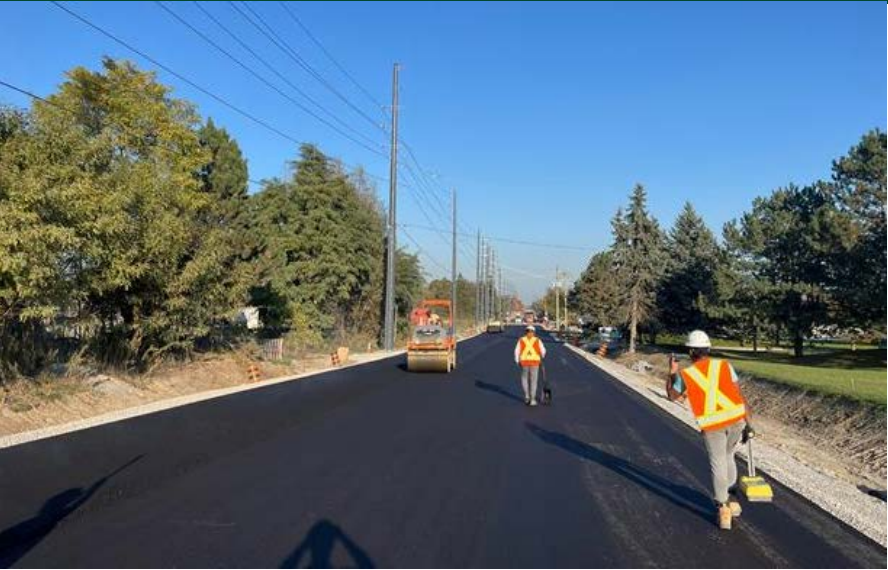
Bethesda Rd Reconstruction (Phase 3)
