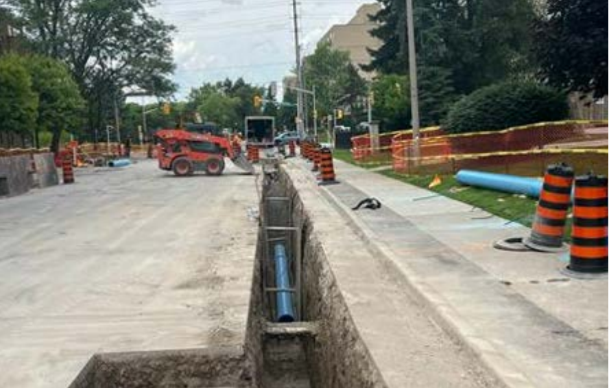
Cedar Ave Watermain Replacement
