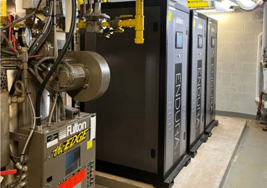
RHCPA (Theatre) Boiler Replacement
