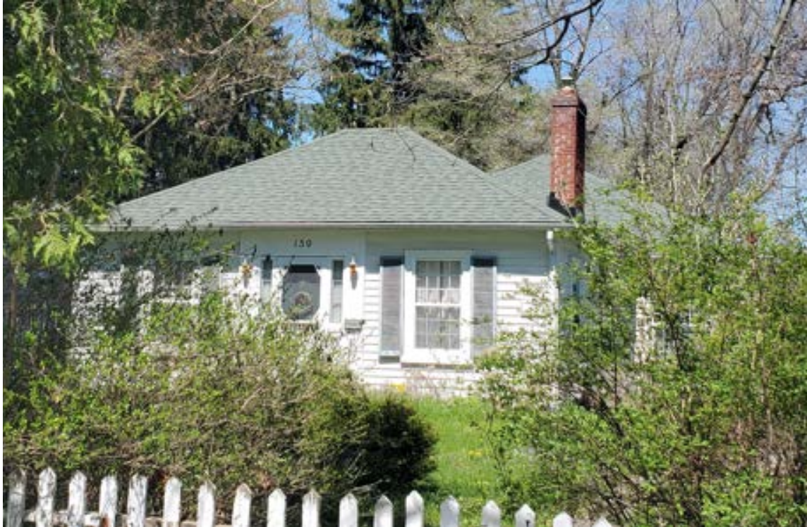
Figure 1 May 2024 photograph of 159 Mill Street showing the historical (south) portion of the building, with a later rear addition visible on the right. All identified heritage attributes are limited to the historical portion of the building, including the house's one-storey massing, hipped roof with wide eaves, symmetrical three bay front façade with a centered doorway, and the appearance of clapboard siding and 12-over-12 windows (Source: HUD 2024).
