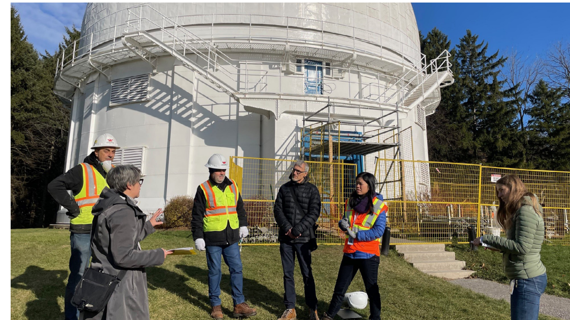
The City and contractors complete a site visit with Parks Canada as part of their support for repairs to the David Dunlap Observatory through the National Cost Sharing Program for Heritage Places. Photo courtesy of Parks Canada.
