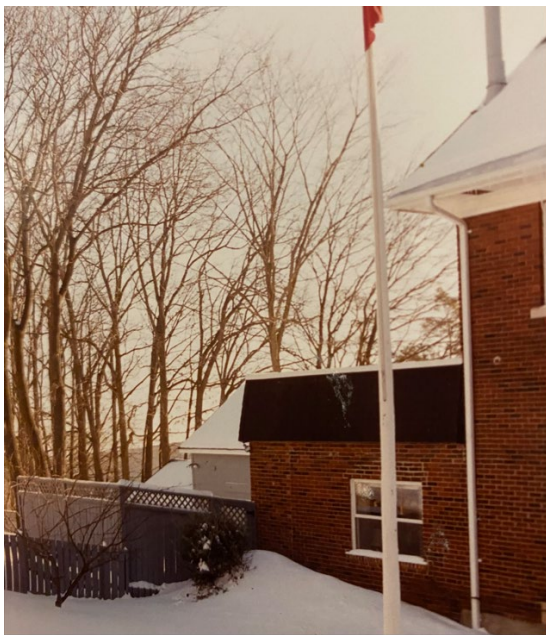
Photo 3. The northern elevation circa 1980. This photo shows the new addition, delineated by the mansard roof. Note that the brick used for this portion of the addition was repurposed from the original rear wall of the house.
