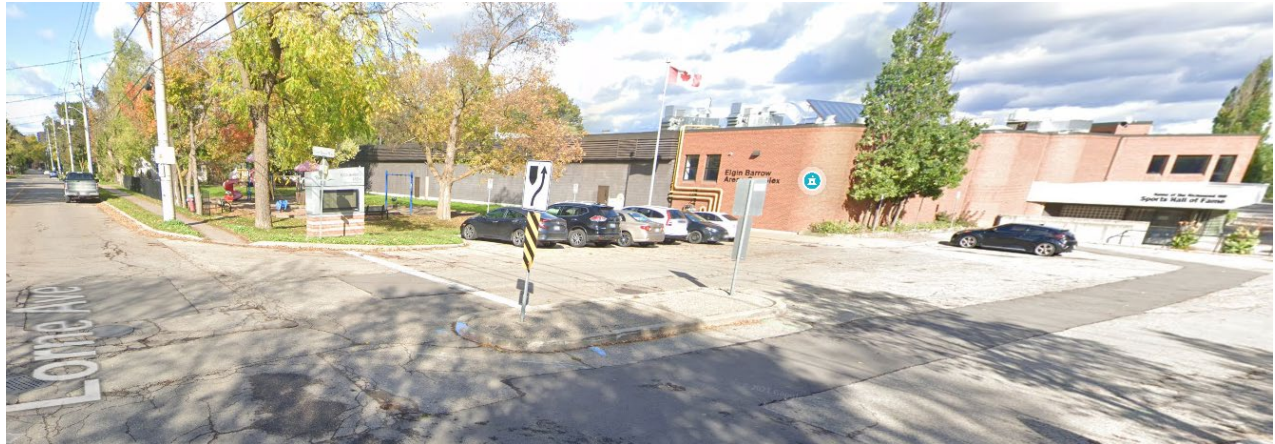
Elgin Barrow Arena Complex at 43 Church Street South, two properties north of the Property (Google Maps)
