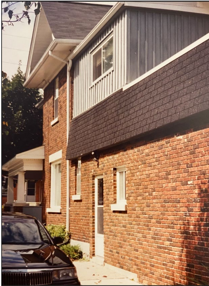
Photo 4. The southern elevation circa 1980s. This photo shows the new mansard roof and grey siding-clad portion of the addition. While original brick from the rear of the house was repurposed to clad the first storey of the addition, all portions of the building immediately to the west of the side door date from the 1970s (as demonstrated by the limit of the original foundation line to the west of the door).
