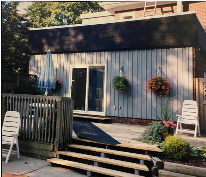
Photo 2. The new eastern (rear) elevation, with addition clad in grey siding
