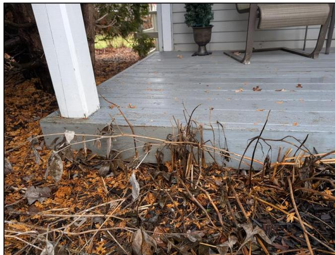
**Figures 2-5 (clockwise from top left):** The existing front porch at 11 Station Road; close-up photos showing that the porch deck rests directly on the ground; water accumulation on basement floor.
