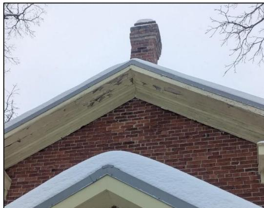
Figures 14-17 (clockwise from top left): cracking paint on verandah post, door, ceiling, and soffit.
