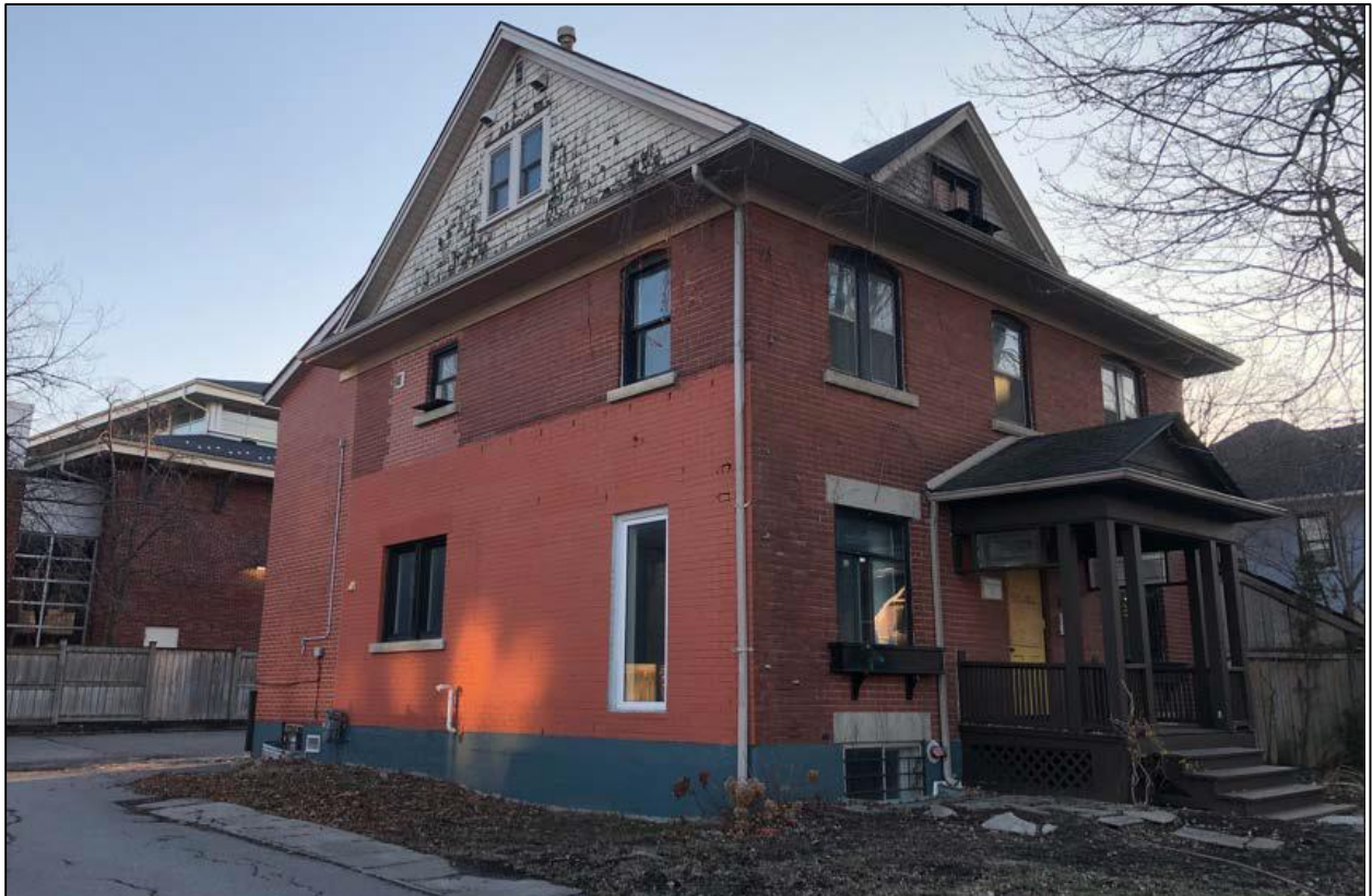
Figure 1: Photograph showing the existing condition of the north and east facades. Note the two-storey brick-clad addition in the rear (City of Richmond Hill, 2023).
