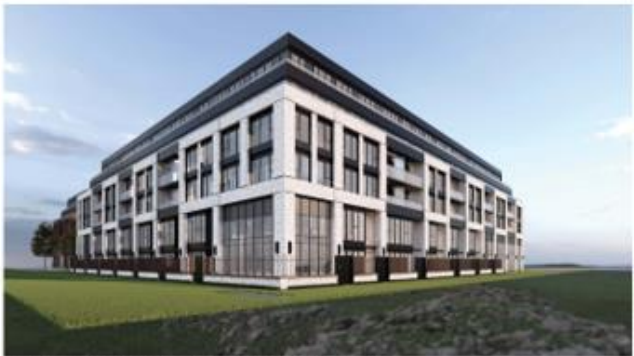
STREET VIEW LOOKING NORTHEAST FROM SOUTHWEST CORNER OF THE SITE
