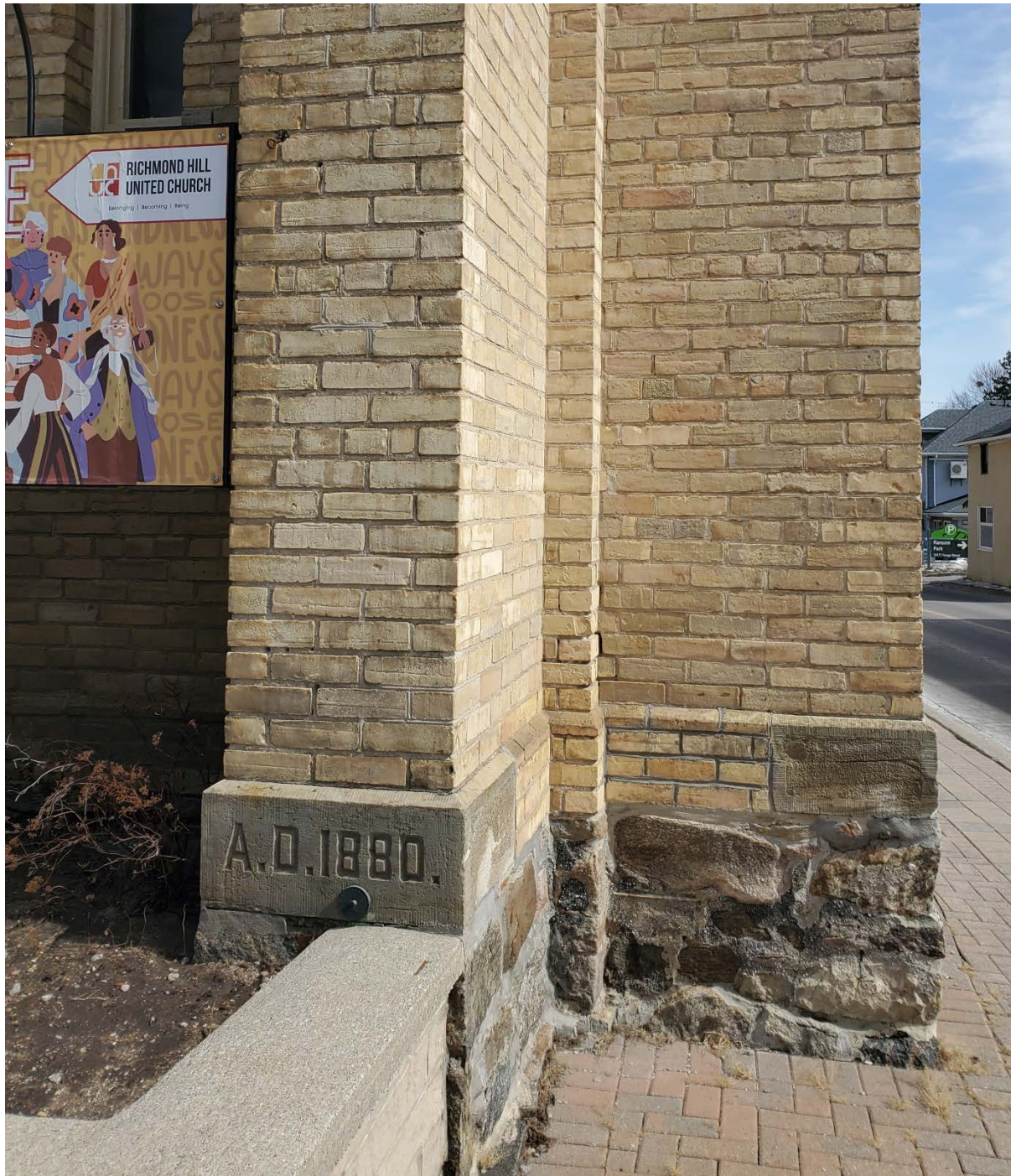
Figure 13 2025 photograph of the Richmond Hill Methodist Church at 10201 Yonge Street looking east at the building's front (west) elevation. Note the date stone inscribed with "A.D. 1880" located on the southwest corner of the building. (Source: HUD 2025)
