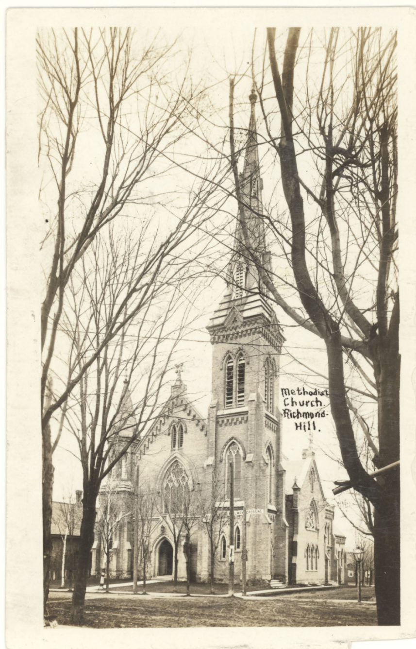
Figure 4 Circa 1910s photograph of the Richmond Hill Methodist Church at 10201 Yonge Street looking northeast, showing the building's front (west) and south elevations. Note the building's square brick towers with octagonal spires, windows with foliated tracery, and prominent location fronting Yonge Street. Also note that the carved stone finial located atop the church gables on the front and side elevations, which have since been removed. (Source: Richmond Hill Public Library Digital Archive)
