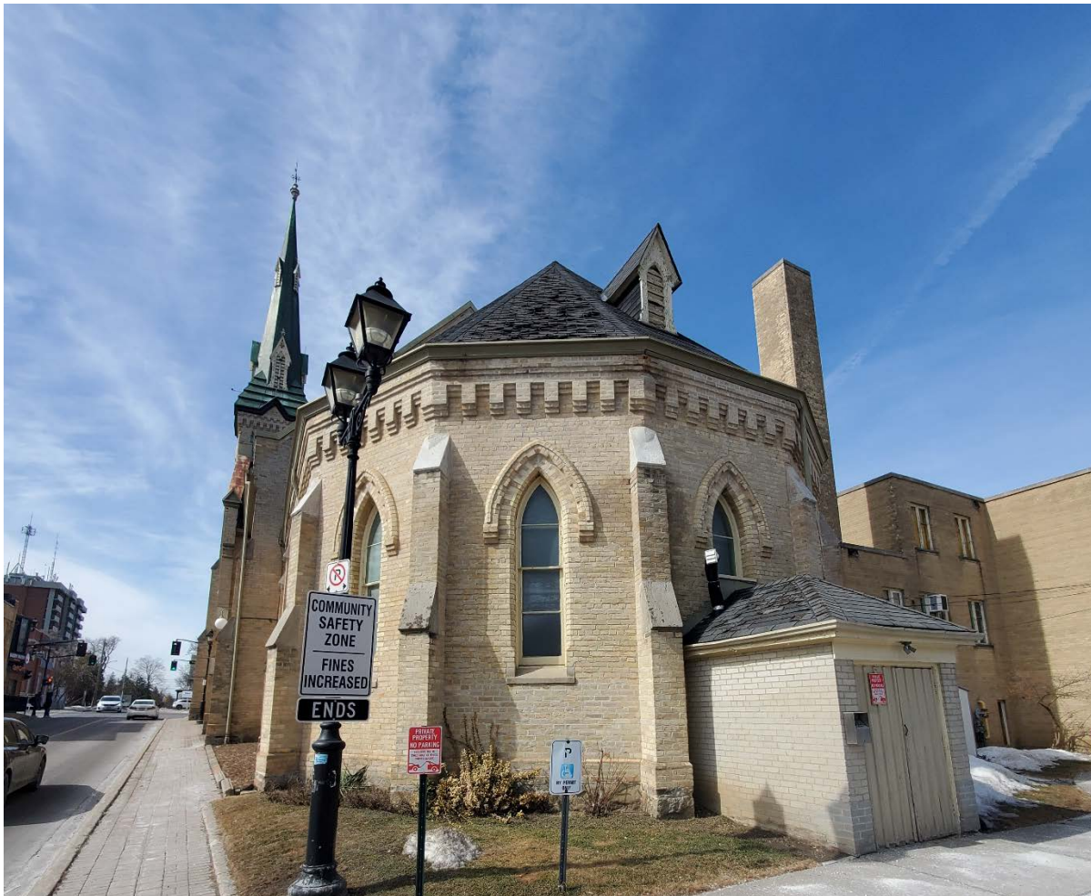
Figure 14 2025 photograph of the Richmond Hill Methodist Church at 10201 Yonge Street looking west at the building's rear (east) elevation. Note the church's polygonal apse, brick buttresses with stone copings, and lancet-arched windows. (Source: HUD 2025)
