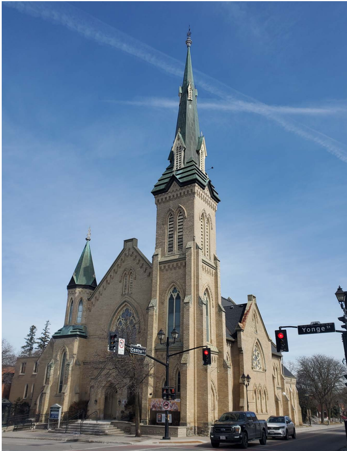
Figure 11 2025 photograph of the Richmond Hill Methodist Church at 10201 Yonge Street looking northwest, showing the church's front (west) and side (south) elevations. Note the church's variety of windows, including lancet-arched stained glass windows with foliated tracery and louvered window units. (Source: HUD 2025)
