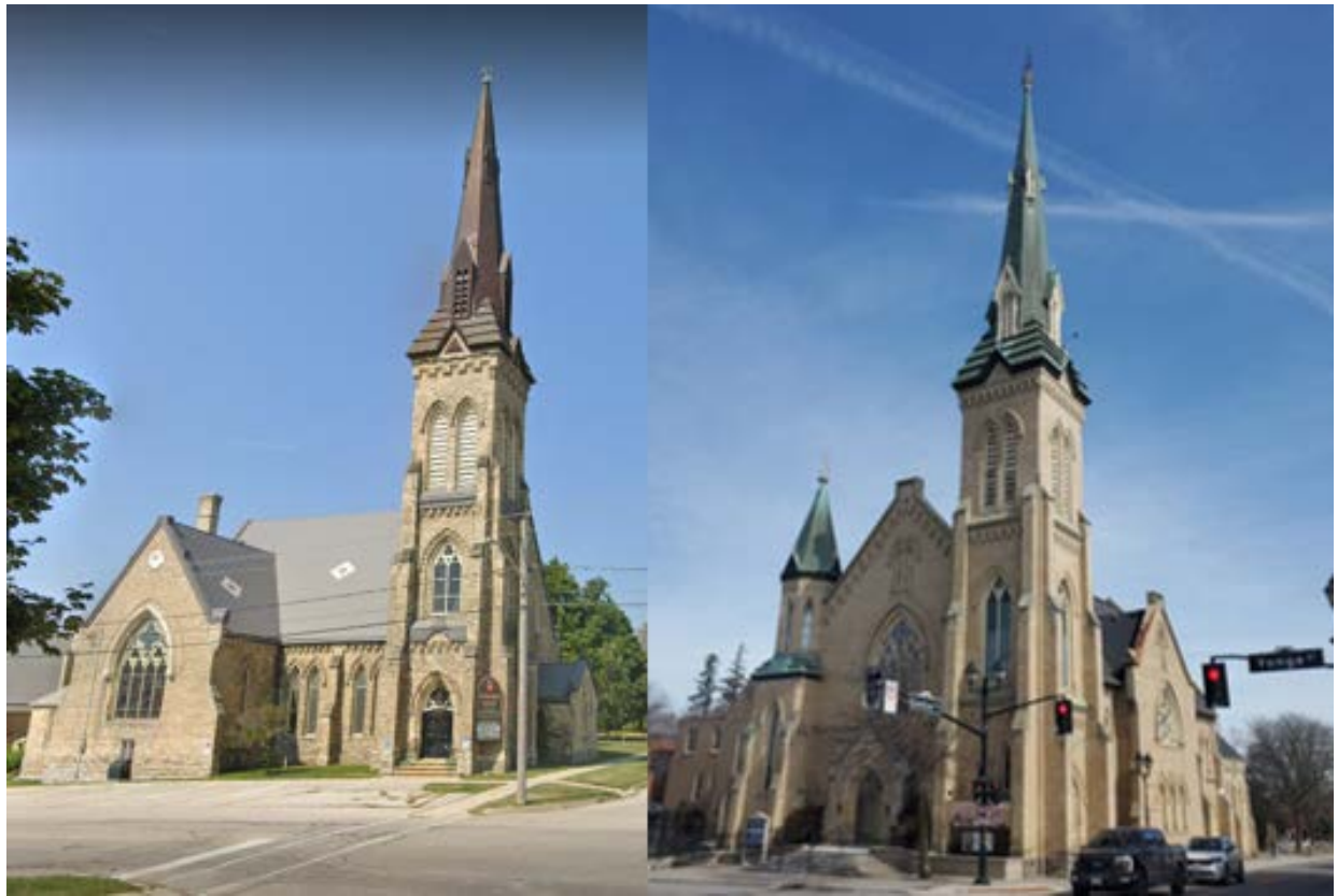
Figure 9 2024 photograph of the St. George United Church in Goderich, Ontario (left) and the Richmond Hill Methodist Church at 10201 Yonge Street (right). Note the similarities between the two church towers, including their tall square massing, buttresses, lancet-arched windows, and steeples with dormer windows. Both churches were designed by architect Charles Walton, who used similar designs for each building. (Source: Google Street View 2024, HUD 2025)
