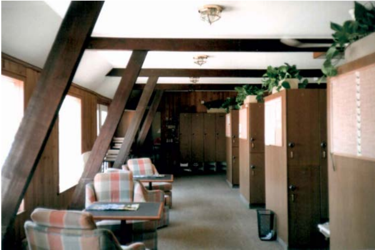
Figure 5 2012 photograph showing the circa 1920s exposed wooden structural elements in the women's locker room at the Summit Clubhouse at 11901 Yonge Street. (Source: Joan Burt Architect, 2012)
