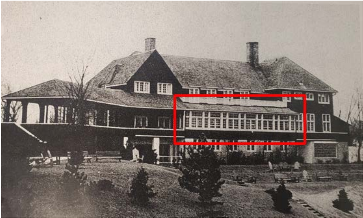
Figure 9 Circa 1940s photograph of the Summit Clubhouse at 11901 Yonge Street looking west, showing the building's rear elevation. Note the ribbon of windows within the structure's enclosed rear verandah (indicated in red), which provided open views of the club grounds to the east. (Source: City of Richmond Hill D12 Folders)
