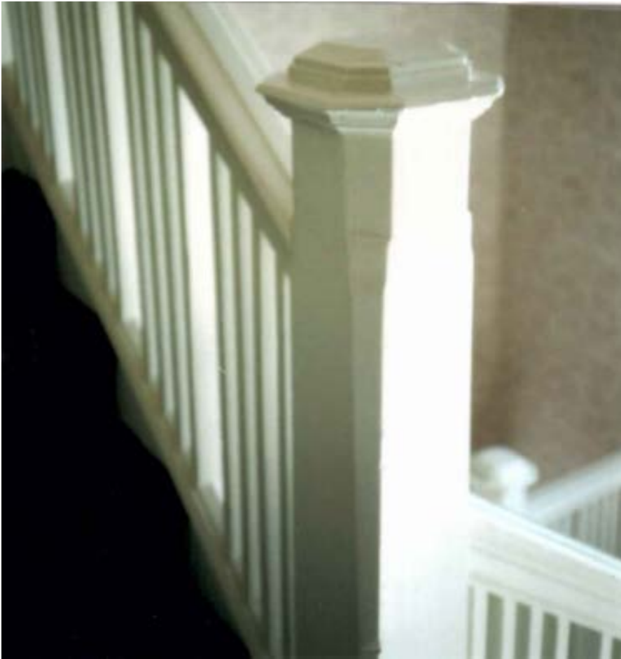
Figure 4 2012 photograph showing the circa 1920s wooden staircase with carved railings and posts at the Summit Clubhouse at 11901 Yonge Street. (Source: Joan Burt Architect, 2012)
