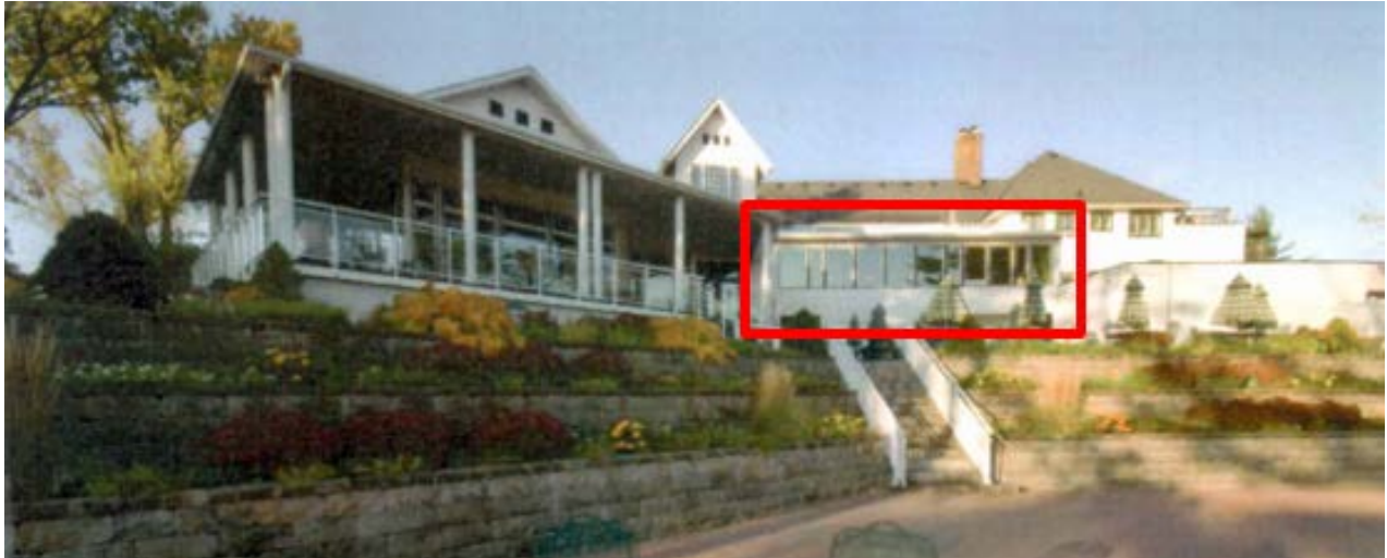
Figure 10 2012 photograph of the Summit Clubhouse at 11901 Yonge Street facing west, showing the building's rear elevation. Note the ribbon of windows within the structure's enclosed rear verandah (indicated in red). Note that while the enclosed verandah has experienced major renovations over the years, the verandah retains the presence of large windows overlooking the golf course, which remains an integral part of the Clubhouse's original design. (Source: Joan Burt Architect, 2012)
