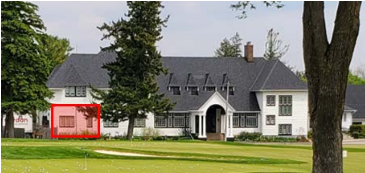
Figure 7 Current photograph of the Summit Clubhouse at 110901 Yonge Street facing east, showing the approximate location of alterations on the building's front (west) façade (indicated in red). Archival documentation shows that the first-storey recessed porch was enclosed circa 1930s – 1940s. (Source: HUD 2024)
