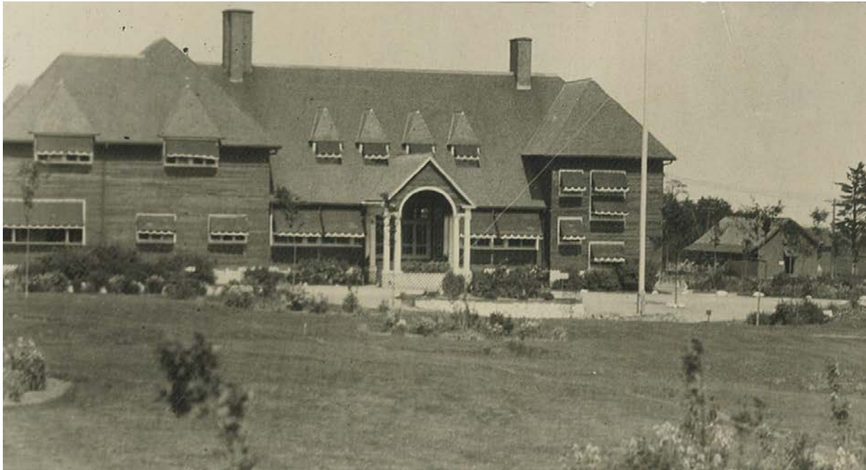
Figure 2 Circa 1930s – 1940s photograph of the Summit Clubhouse at 11901 Yonge Street looking east. Note the building's elongated irregular footprint, steeply-pitched hipped roof with wide eaves and elongated dormers, asymmetrical fenestration pattern, and projecting front-gable portico. Also note that the original first-floor recessed porch at the building's northwest corner has been enclosed by this time. (Source: Toronto Public Library Digital Archives)
