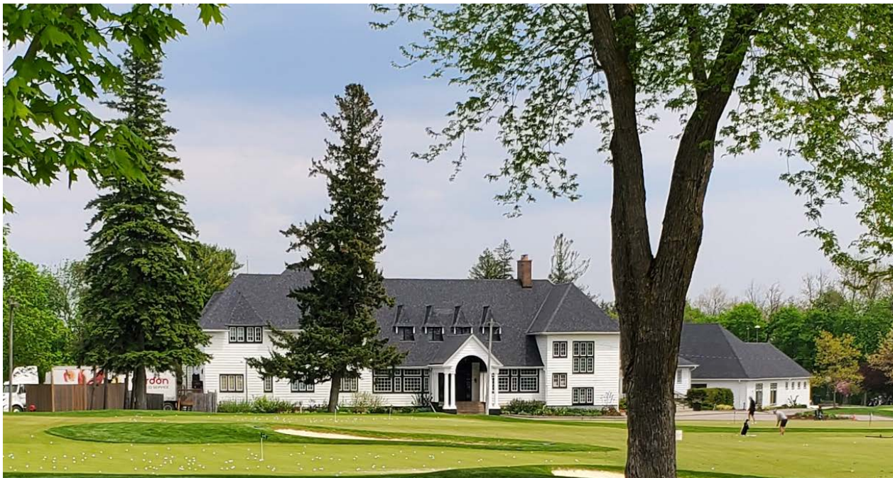
Figure 8 Current photograph of the Summit Clubhouse at 11901 Yonge Street facing east, showing the building's principal (west) elevation. Note the structure's irregular footprint, steeply-pitched hipped roof with wide eaves and elongated dormers, asymmetrical fenestration pattern, and projecting front-gabled portico. (Source: HUD 2024)
