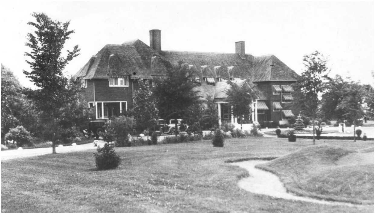
Figure 1 Circa 1920s – 1930s photograph of the Summit Clubhouse at 11901 Yonge Street looking southeast. Note the building's elongated irregular footprint, steeply-pitched roof with wide eaves and elongated dormers, asymmetrical fenestration pattern, and picturesque circular driveway. Also note that at this time the building featured a recessed porch at its northwest corner, which was later enclosed (Source: Richmond Hill Public Library Digital Archive)
