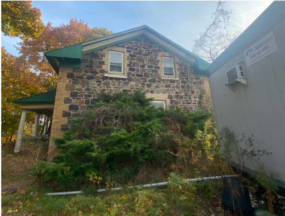
Figure 6 Current photograph looking east, showing the west (side) elevation of the Peter Heise House at 1591 Elgin Mills Road East. Note the low-pitched side-gabled roof with wide return eaves, buff brick quoining at corners and around windows, and the variegated fieldstone cladding. (Source: HUD, 2024)
