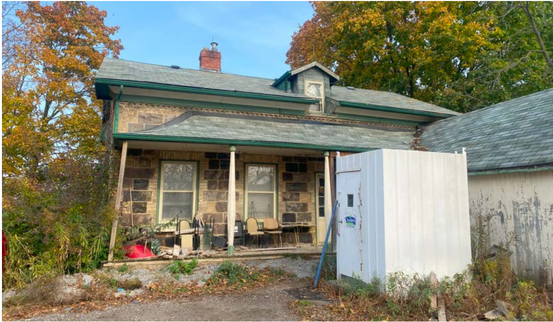
Figure 8 Current photograph looking north, showing the south elevation of the Peter Heise House at 1591 Elgin Mills Road East. Note the low-pitched side-gabled roof with later dormer window, large, squared stone cladding, buff brick quoining, sawtooth banding below the eaves, asymmetrical four-bay composition, and full-façade bellcast-roofed verandah on tapered octagonal posts. The summer kitchen addition can be seen on the far right of the image. (Source: HUD, 2024)
