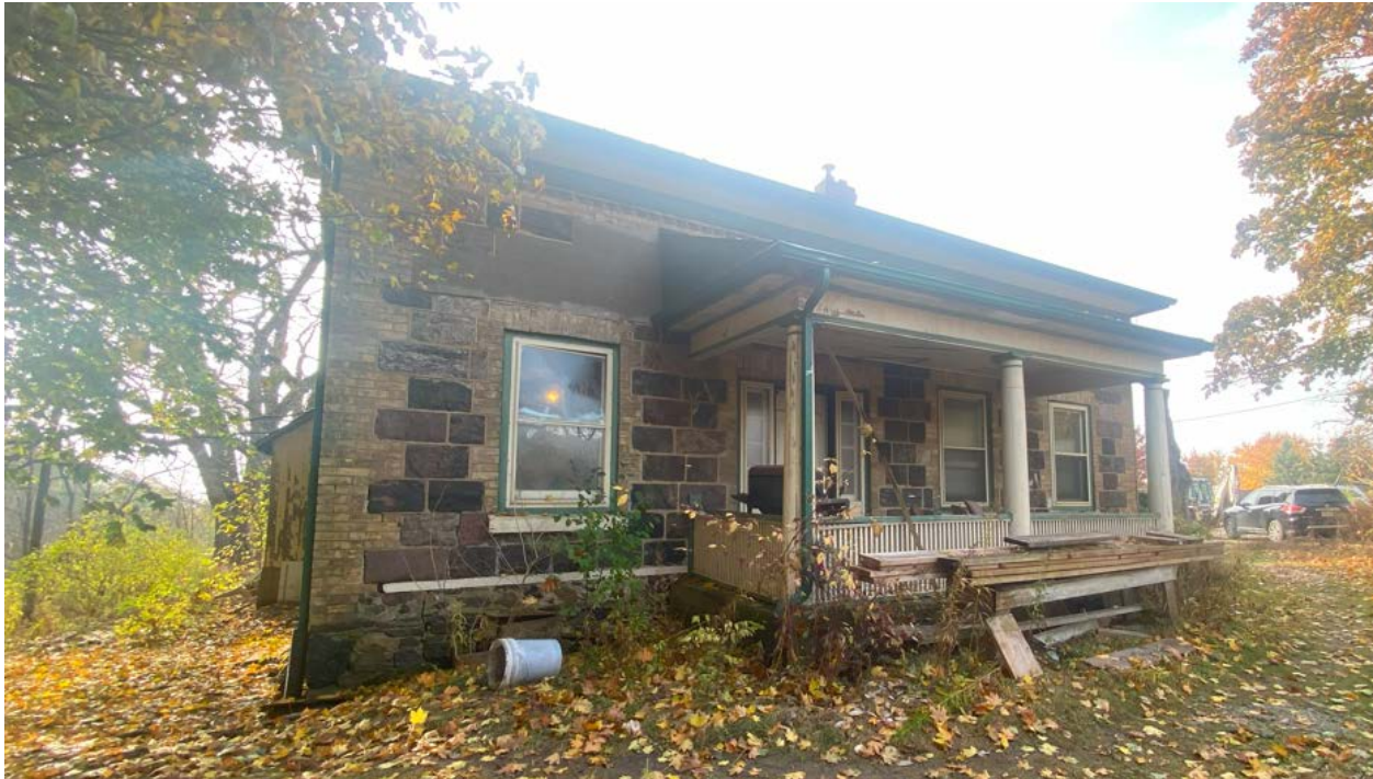
Figure 4 Current photograph looking southeast, showing the north elevation of the Peter Heise House at 1591 Elgin Mills Road East. Note the low-pitched side-gabled roof, large, squared stone cladding, buff brick quoining and banding, asymmetrical four-bay composition, and the classical doorcase with sidelights and a wooden door. Note also the presence of a wooden beam spanning the elevation at ground-floor level and parging below the eaves, indicating an earlier full-façade verandah. (Source: HUD, 2024)
