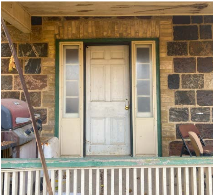
Figure 5 Detailed photograph of the classical doorcase on the north elevation of the Peter Heise House at 1591 Elgin Mills Road East. Note the buff-brick quoining, sidelights, and six-paneled wooden door. Also note the large, squared stone cladding on this elevation. (Source: HUD, 2024)
