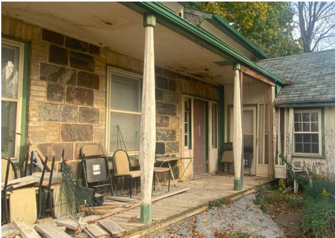
Figure 9 Detailed photograph looking northeast, showing the tapered octagonal columns and classical doorcase on the Peter Heise House's south elevation. (Source: HUD, 2024)
