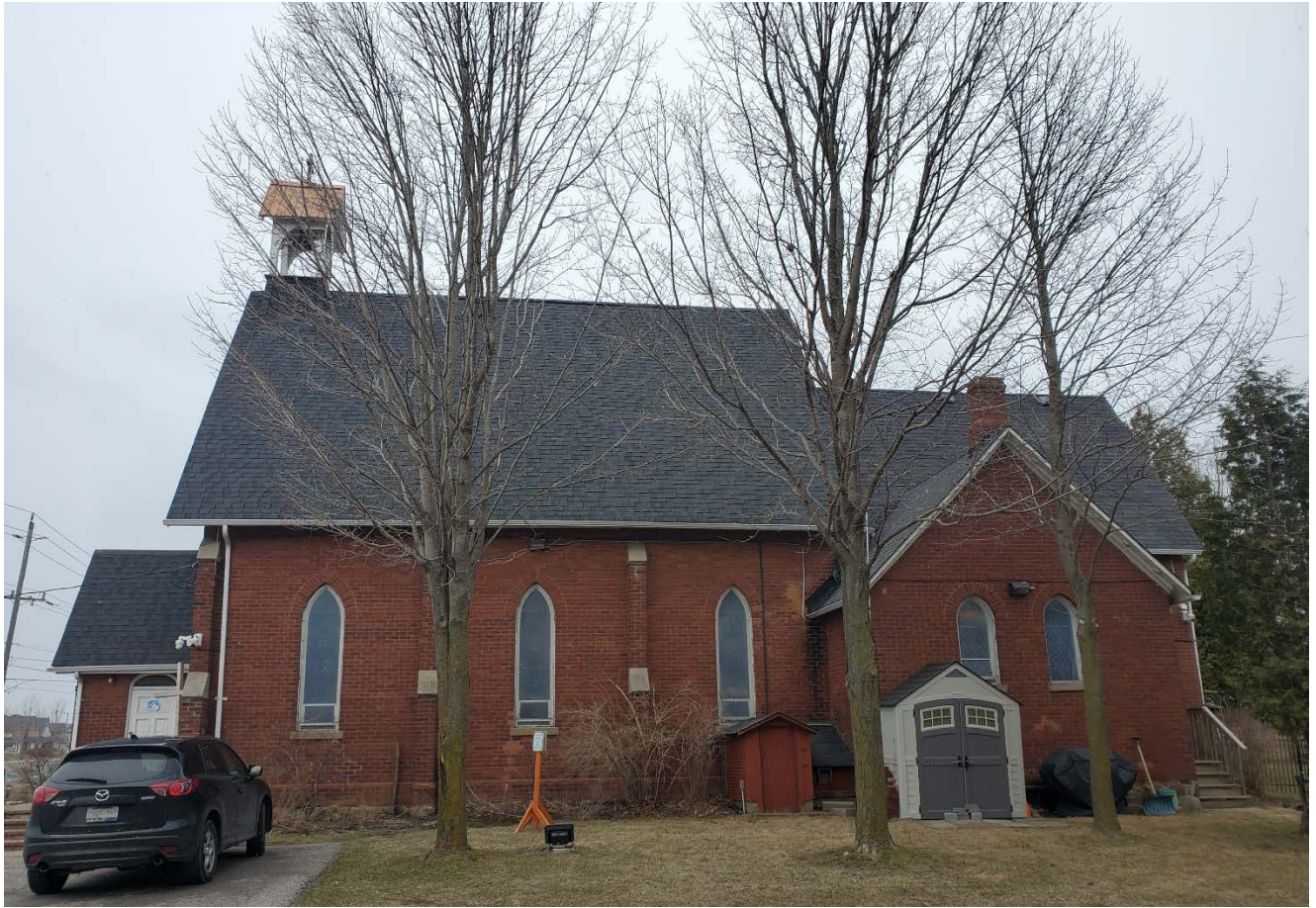
Figure 14 2025 photograph of the St. John the Baptist Church at 12125 Yonge Street looking north, showing the Main Church's south (side) elevation. Note the building's brick buttresses with stone copings. Also note the cross-gable-roofed chancel and vestry projecting from the rear of the chapel, visible on the right of the image. (Source: HUD 2025)
