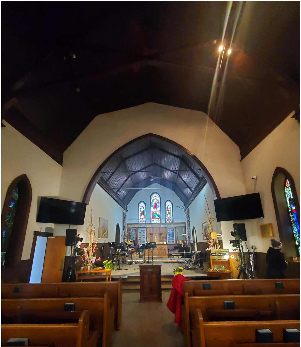
Figure 16 2025 interior photograph of the St. John the Baptist Church at 12125 Yonge Street looking east towards the chancel. Note the vaulted ceilings with exposed wooden rafters of both the nave and the chancel, the lancet-arched chancel located at the east end of the church, and the stained glass lancet-arched tripartite window on the east wall of the chancel. (Source: HUD 2025)
