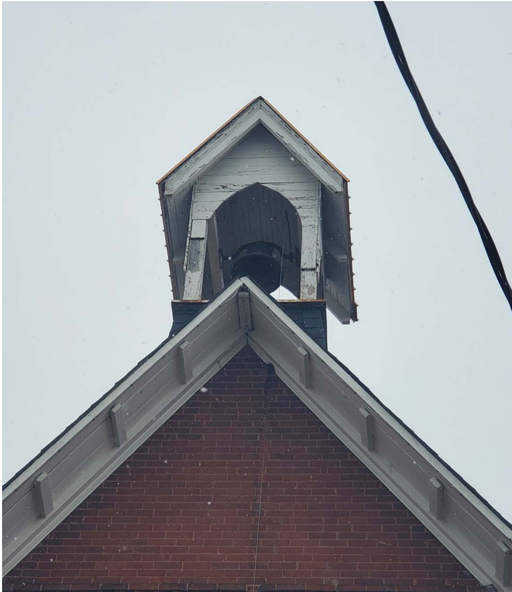
Figure 12 2025 detail photograph of the St. John the Baptist Church at 12125 Yonge Street looking east, showing the church's gable-roofed belfry with lancet-arched openings. (Source: HUD 2025)
