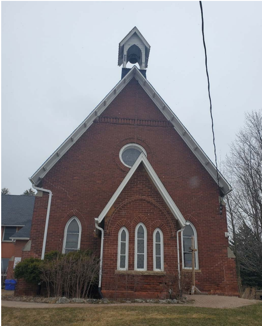
Figure 13 2025 photograph of St. John the Baptist Church at 12125 Yonge Street looking east, showing the chapel's front (west) elevation. Note the church's simple and symmetrical front façade, steeply-pitched gabled roof with belfry and bracketed eaves, lancet-arched and roundel stained glass windows, and decorative brick banding. (Source: HUD 2025)
