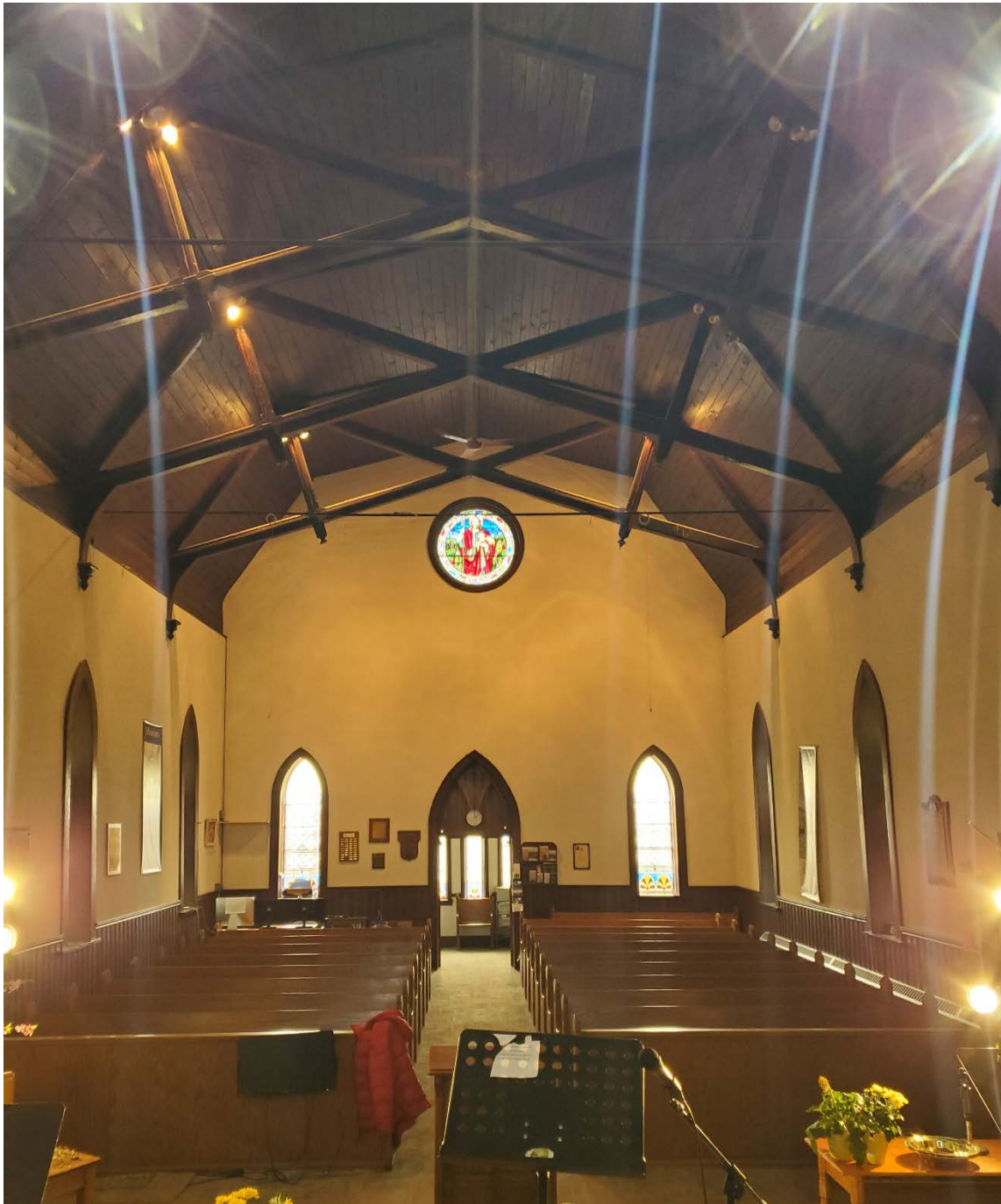
Figure 17 2025 interior photograph of the St. John the Baptist Church at 12125 Yonge Street looking west, showing the west wall of the nave. Note the vaulted ceiling with exposed wooden rafters. (Source: HUD 2025)
