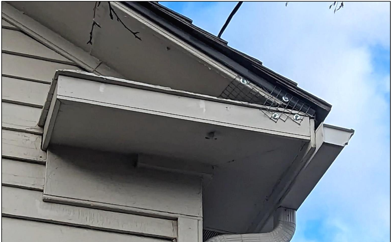
Figure 2: Area on west elevation showing deterioration and “alligatoring” paint.
