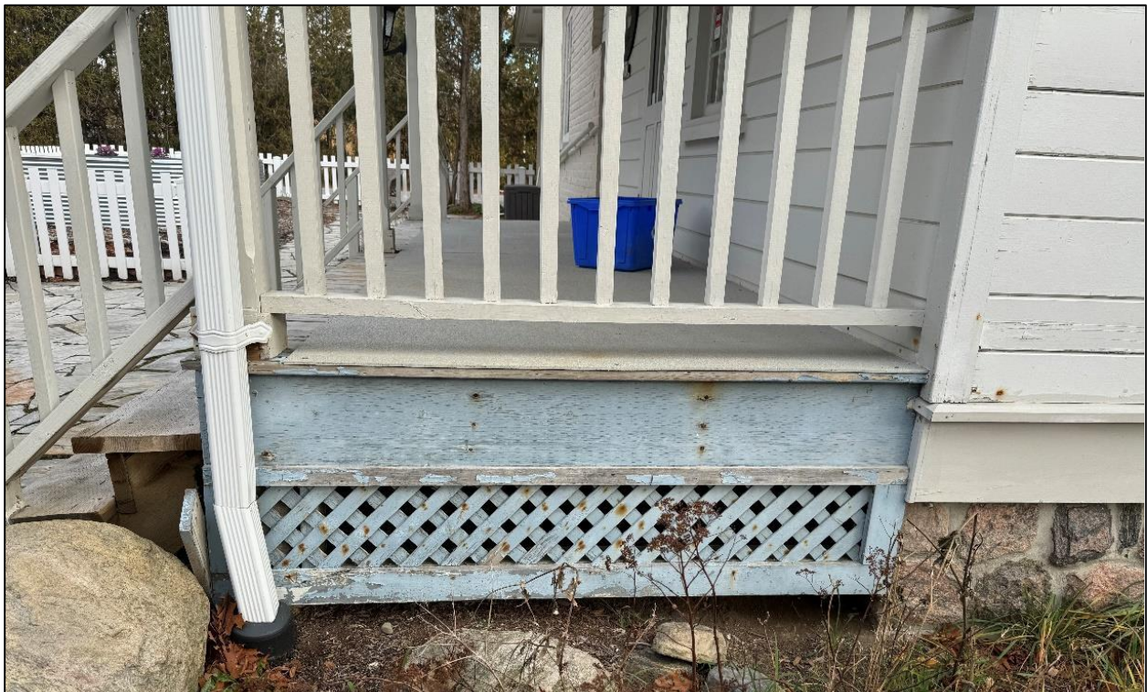
Figure 6: Skirting board showing areas of peeling paint, rusting nails.
