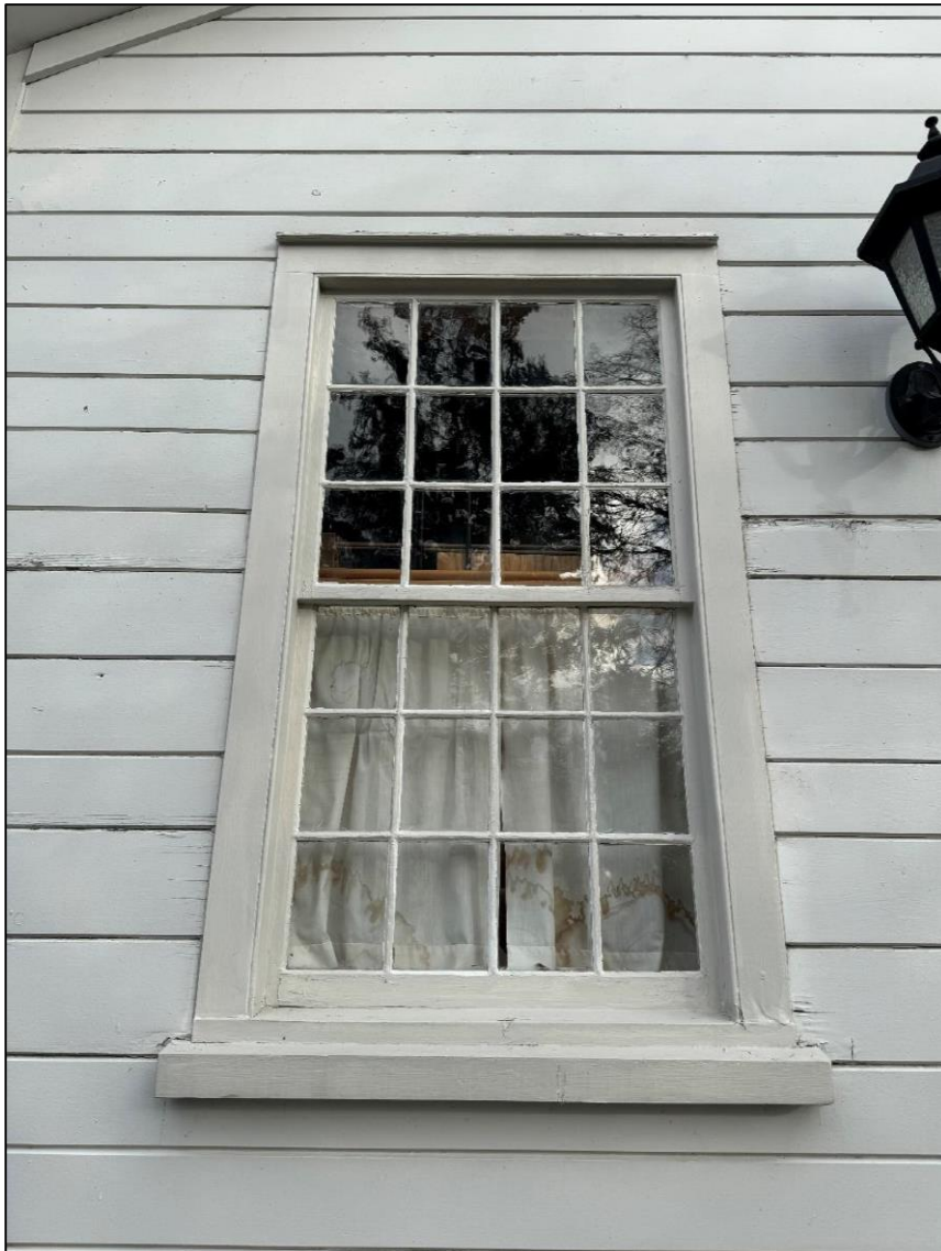
Figure 3: Typical window on south elevation showing areas of cracking, peeling paint.
