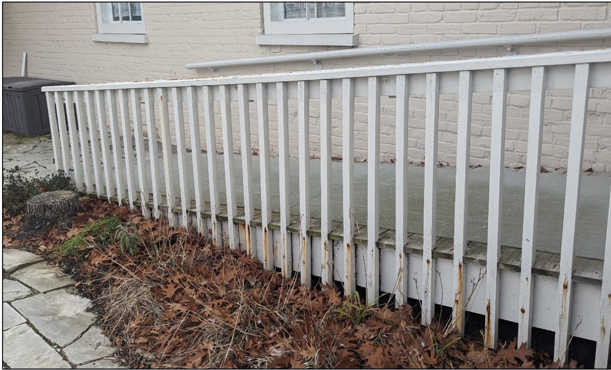
Figure 8: Ramp along northern façade showing flaking paint, rusted nails, degrading wooden planks.
