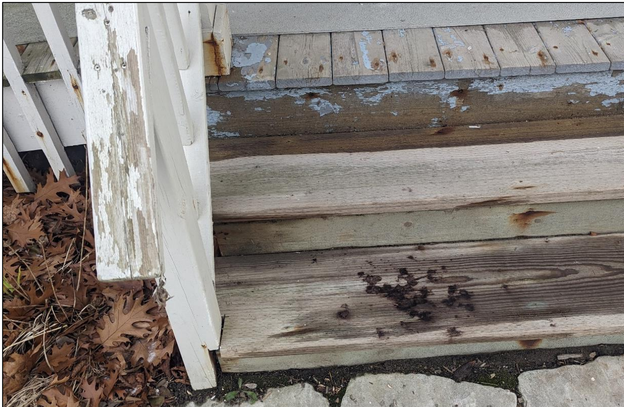
Figure 9: Wooden steps and porch showing degraded wood, chipping paint, rust stains.
