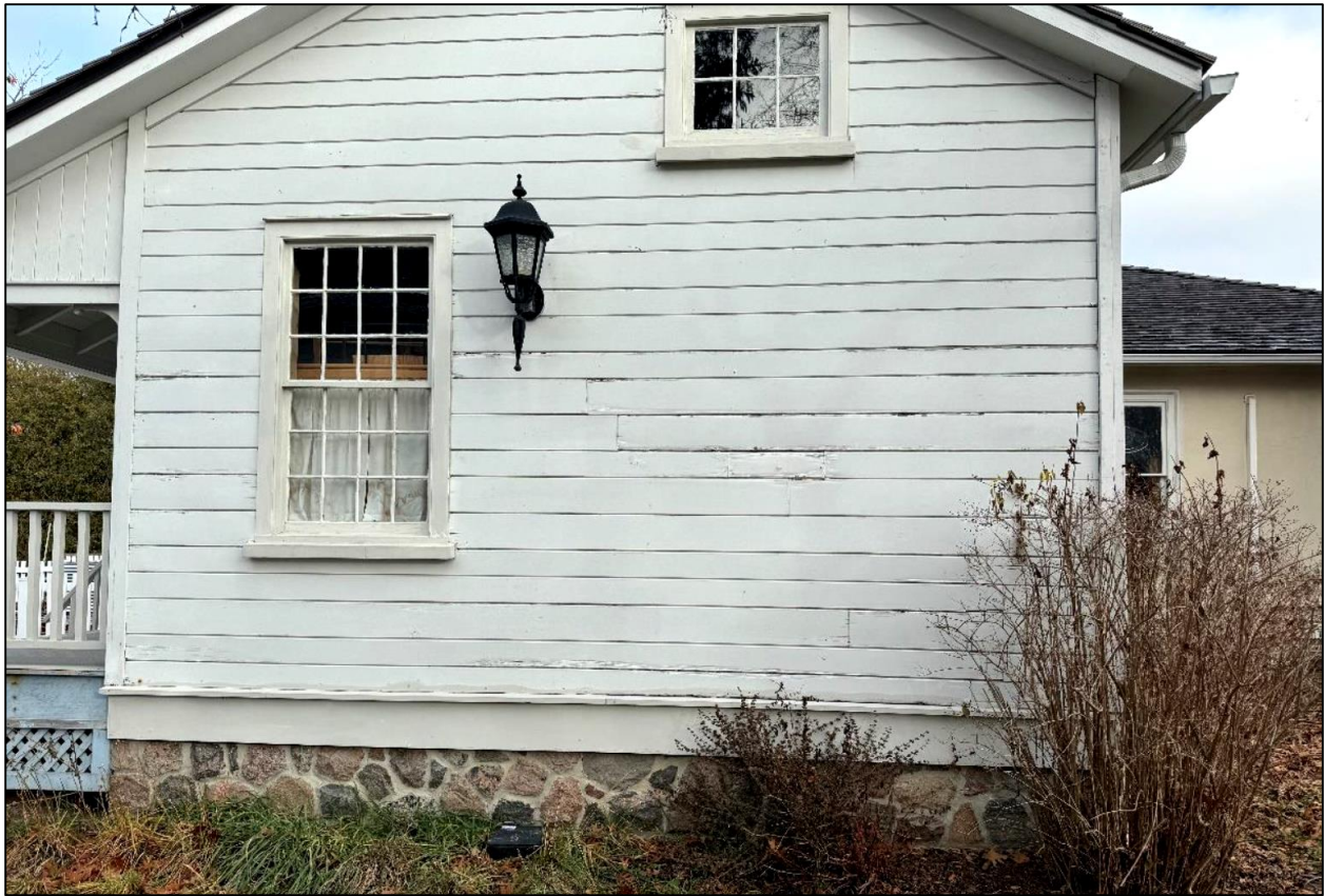
Figure 4: Siding on west elevation showing areas of wood rot and failing paint.
