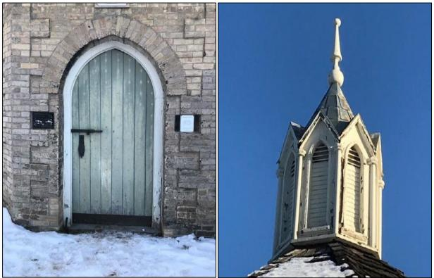
Figures 18, 19: Pointed archway and door (left), and ventilator (right) showing peeling paint and deterioration.
