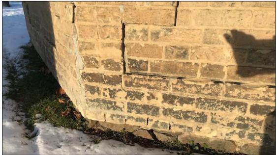
Figure 17: Typical damage to bricks on the exterior of the Octagonal Vault.
