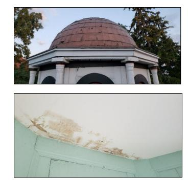
**Figures 2-4:** Exterior of the cupola showing degradation (left), with the roof (top) showing flaking tiles and water damage (bottom).
