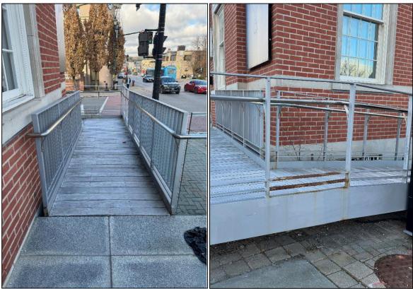
Figure 6 and 7: Planks sowing areas of damage (left), rusted metal railings (right).
