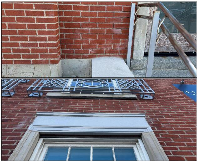
Figures 8 and 9: Examples of efflorescence on the front façade.
