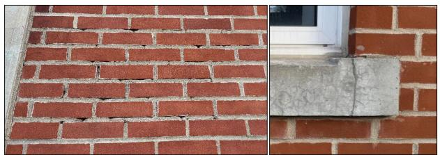
Figures 10 and 11: Examples of degraded mortar (left), cracks on window sill (right).
