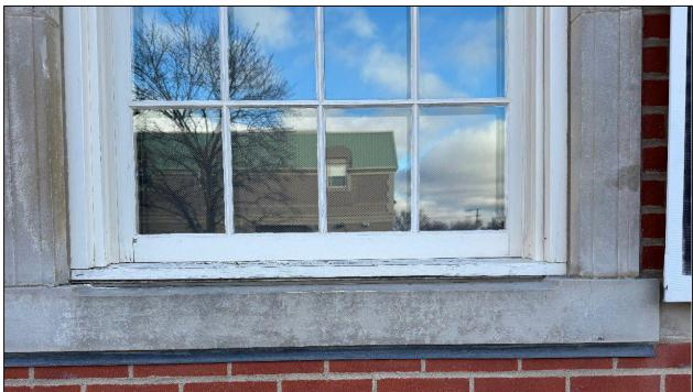
Figure 5: Window showing cracks, degraded paint.
